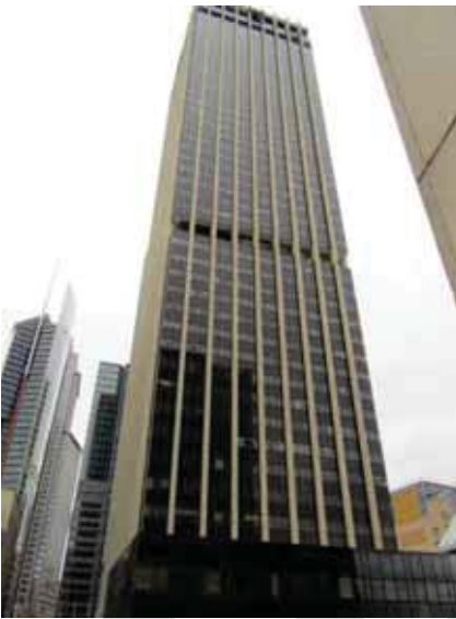
VIEW SOUTH TO 50 BRIDGE STREET (AMP CENTRE)
