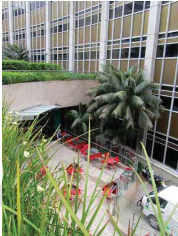
VIEW OF THE PODIUM/ PLAZA AND INTERFACE WITH THE SUBJECT 33 ALFRED STREET
