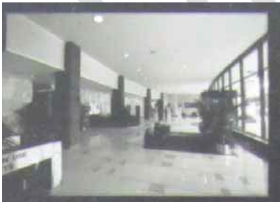
THE MAIN LOBBY VIEW WEST SHOWING ORIGINAL FINISHES SOURCE: CLIVE LUCAS STAPLETON/ ARCHIVAL RECORDING FOR CONDITION OF CONSENT D99/01004
