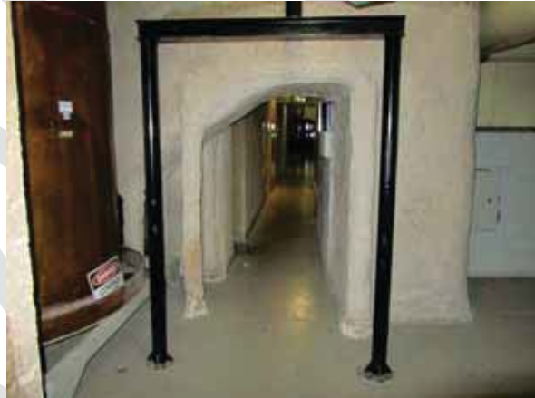
GENERAL PLANT VIEW INCLUDING ONE OF THE FLUSHING TANKS
