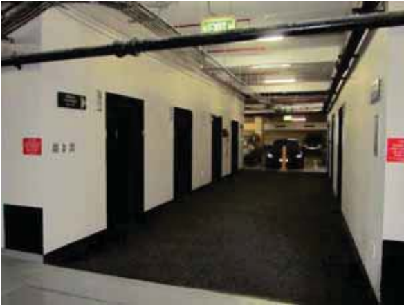
BASEMENT LIFT LOBBY
