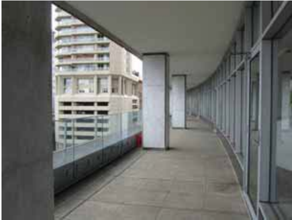
ORIGINAL CURTAIN WALLING, MARBLE CLADDING, PAVING AND BALUSTRADE
