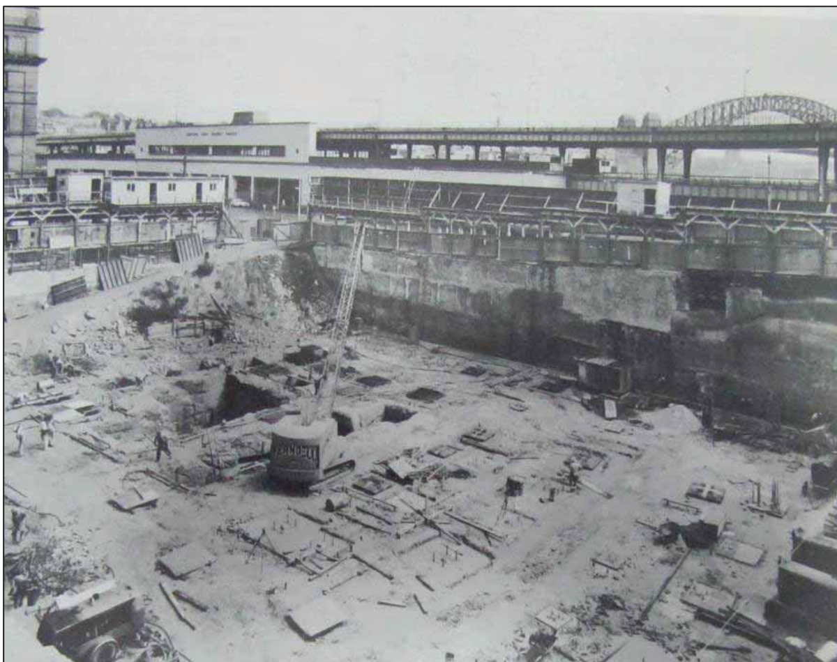
EXCAVATION UNDERWAY AT THE SITE OF THE AMP BUILDING, 1 MARCH 1960
