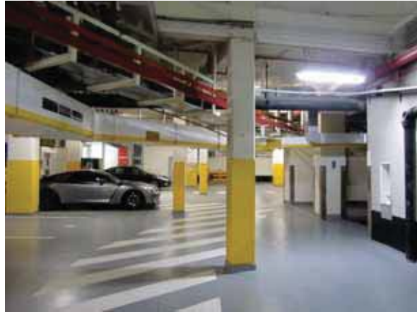
CARPARK VIEW WEST WITH THE SERVICE CORE AT RIGHT
