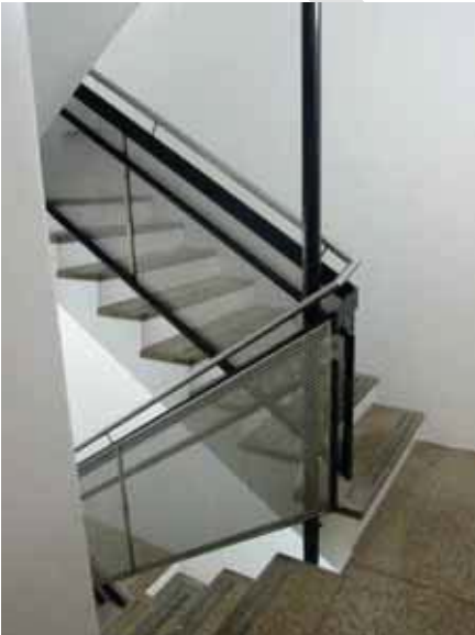
VIEW OF TERRAZZO FIRE STAIR FROM LEVEL 5 (INDICATIVE VIEW FOR COMMERCIAL FLOORS)
