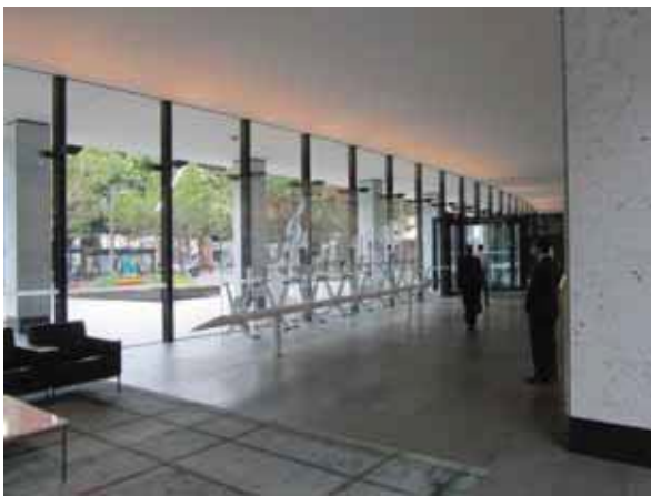
MAIN LOBBY VIEW NORTH EAST SHOWING THE CURVED CURTAIN WALL GLAZING AND TORCH DISPLAY
