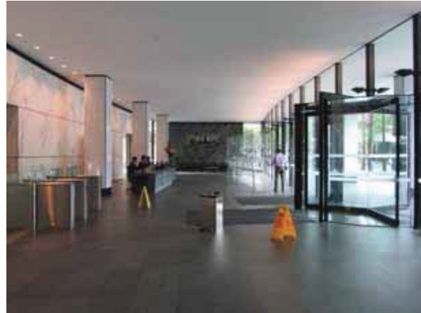
MAIN LOBBY VIEW WEST SHOWING THE NEW REVOLVING DOORS, REFURBISHED FLOOR AND CEILINGS AND ORIGINAL MARBLE FINISHES
