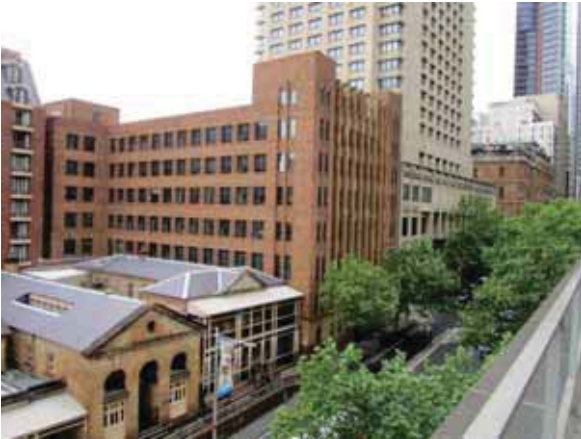
VIEW SOUTH ALONG PHILLIP STREET SHOWING THE STATE HERITAGE LISTED JUSTICE AND POLICE MUSEUM AND ADJACENT HERITAGE ITEMS
