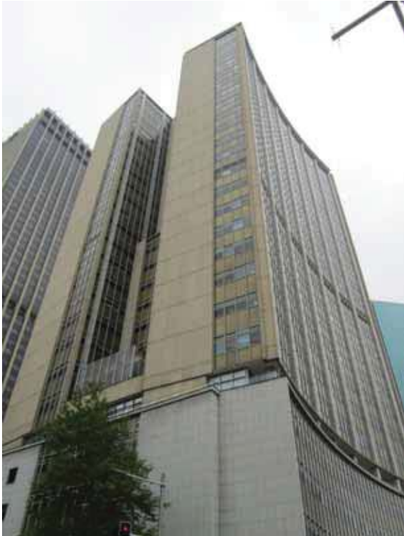
THE TWO AMP TOWERS FROM PHILLIP STREET (33 ALFRED STREET (AT RIGHT) AND PART VIEW OF 50 BRIDGE STREET (LEFT))
