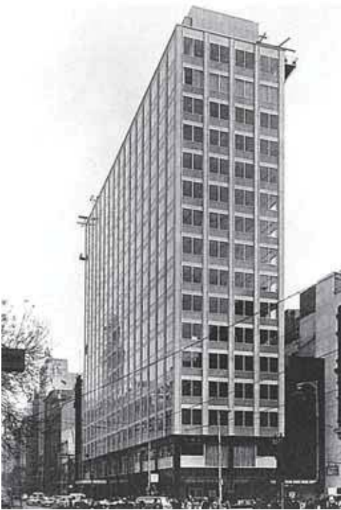
FIGURE 72 – SUN ALLIANCE BUILDING, 1965
